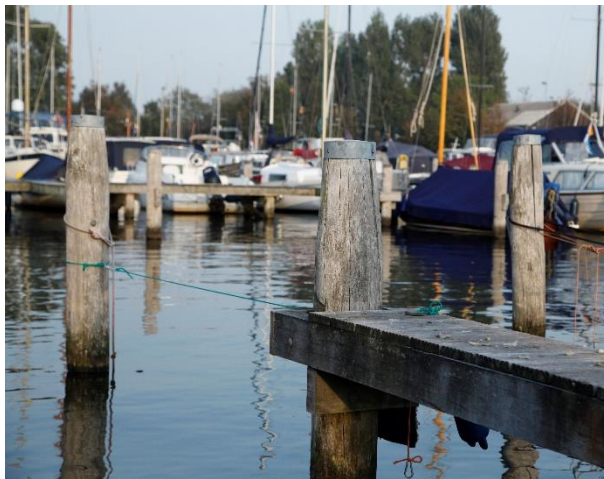
Piling as of 2009, picture of 2018 Source: Mark van Benthem, Stichting Probos
